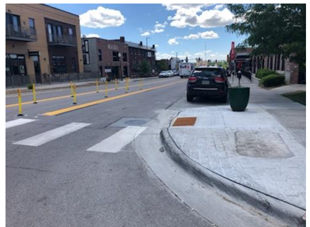
Figure 15. Curb Extension in Blackstone, Omaha (Source Keep Omaha Moving)
