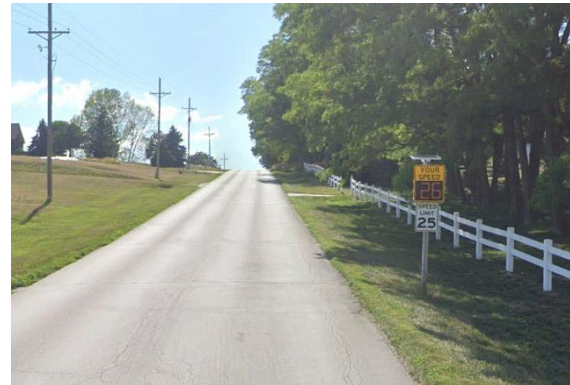
Figure 11. Existing Your Radar Speed Sign on Westbound Clay Street
