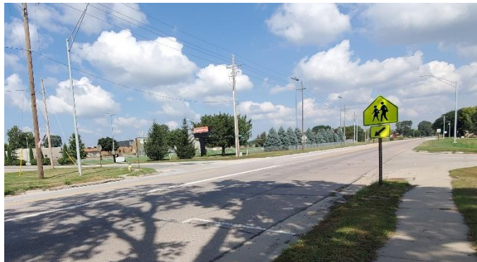
Figure 7. Uncontrolled School Crossing on Northbound US-75
